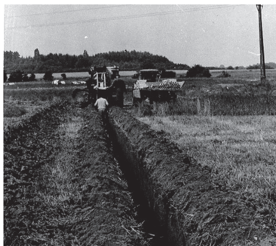
1: Historical photo of construction of a hydromelioration system – example of grooving source: Author's archive
